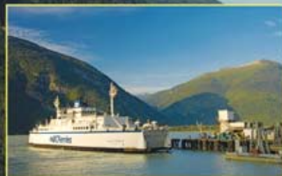
Bella Coola Wharf & Ferry Terminal
